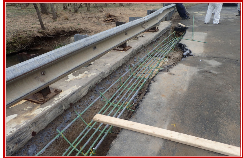
DURING ARCH REPAIR
