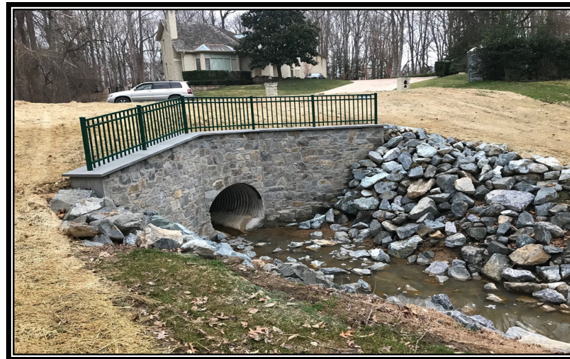
AFTER CULVERT REPAIRS
