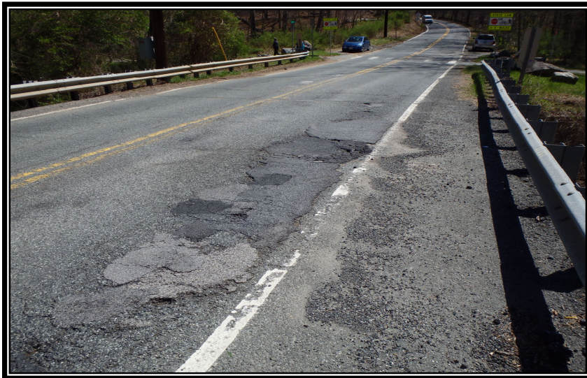
PAVEMENT SPALLING AND LOOSE CORRUGATED METAL DECK PLANKS
