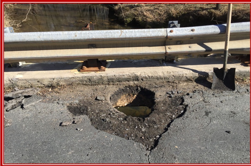
BEFORE ARCH REPAIR
