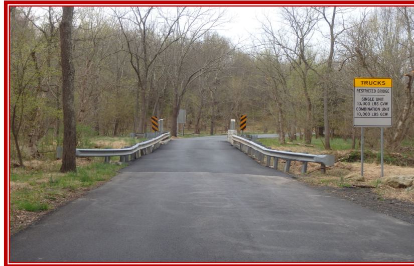
AFTER ARCH REPAIR
